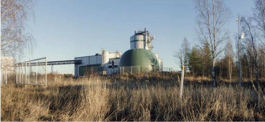
Figure 23: Biogas facility in Mäkikylä, Kouvola
