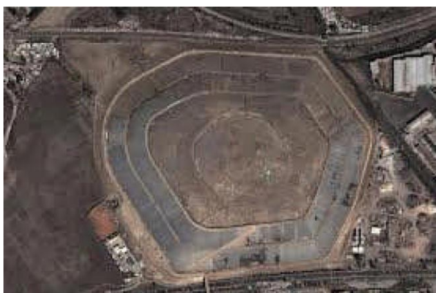
Figure 64: Rehabilitation of OuedSmar landfill
