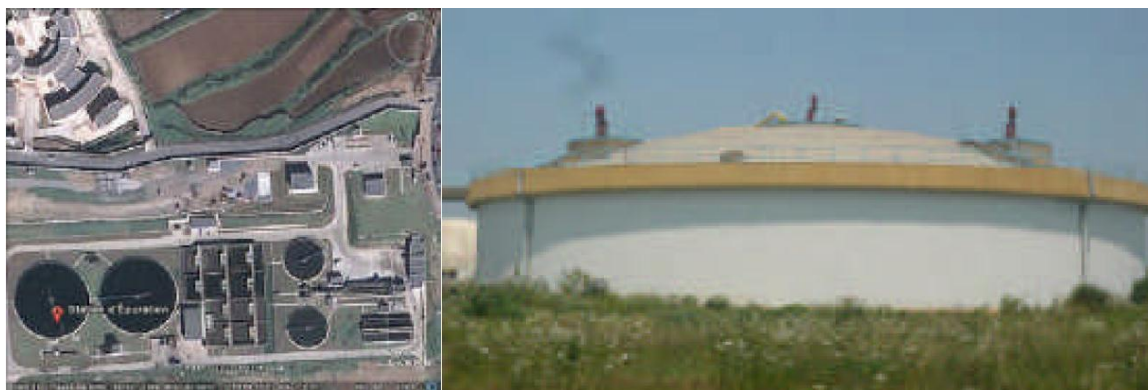
Figure 65: Waste water treatment plant Baraki with the digester
